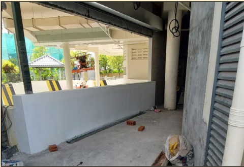
(Pic. 1) Kitchen Corridor
