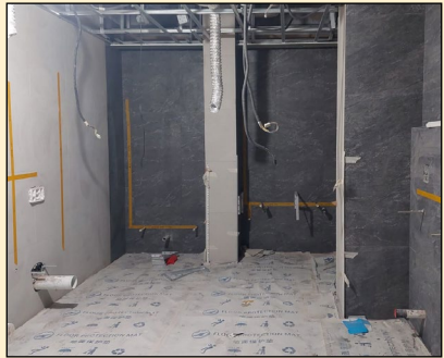
(Pic. 2) Level 1 Toilet
