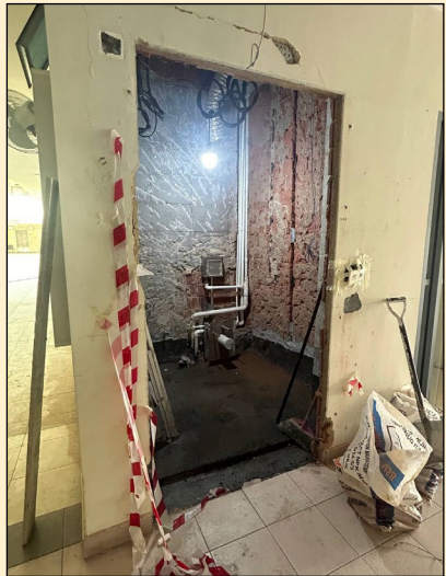
(Pic. 3) Level 1 Handicap Toilet
